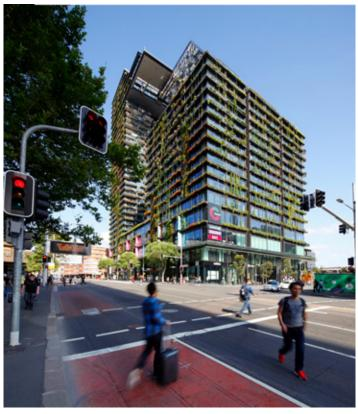
The residential tower at One Central Park features a trigeneration system, water recycling plant and green walls irrigated with recycled water
